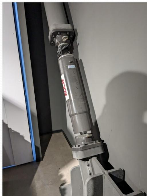
▲(左圖)鋼板阻尼器Steel Panel Damper (SPD) 實況裝安裝
